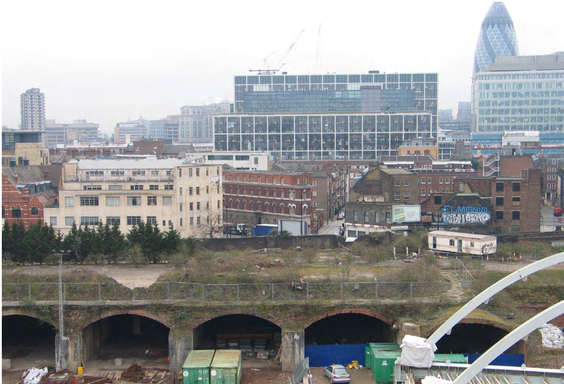
Fig.46: View of Bishopsgate Goods Yard, facing south
